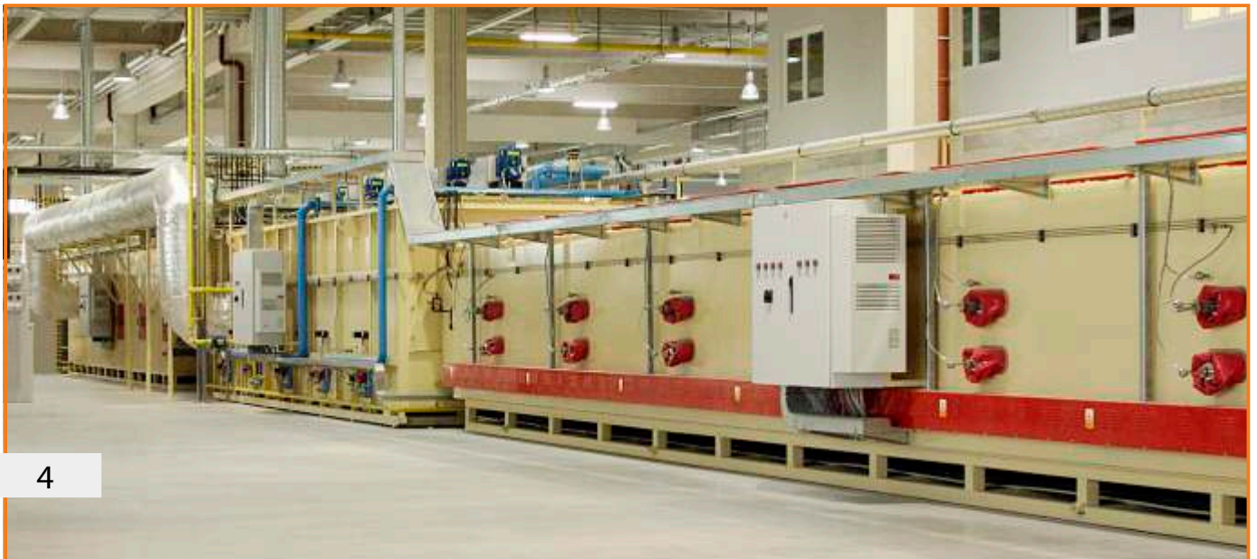
Continuous operating CAB furnace with five preheat and seven braze zones
